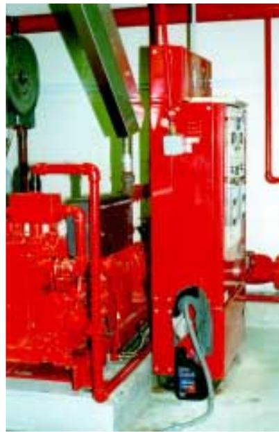
**Figure 2 Unrestrained control cabinet for diesel powered emergency sprinkler pump**
