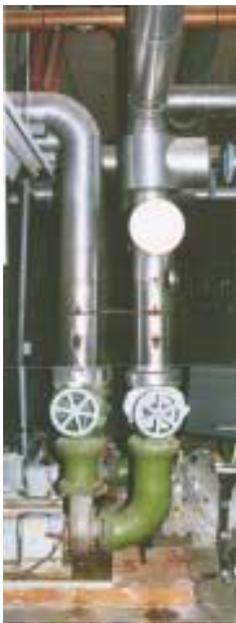
**Figure 1 Insufficiently braced pipe work above pumps**
